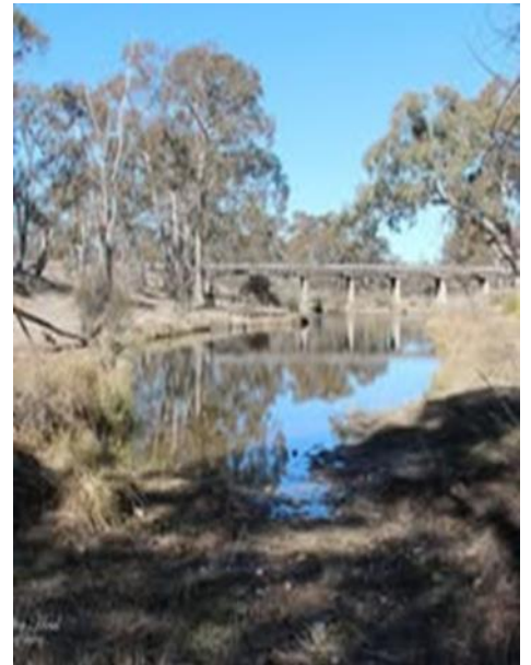
The now removed (in 2021) railway bridge over the Deepwater River.
